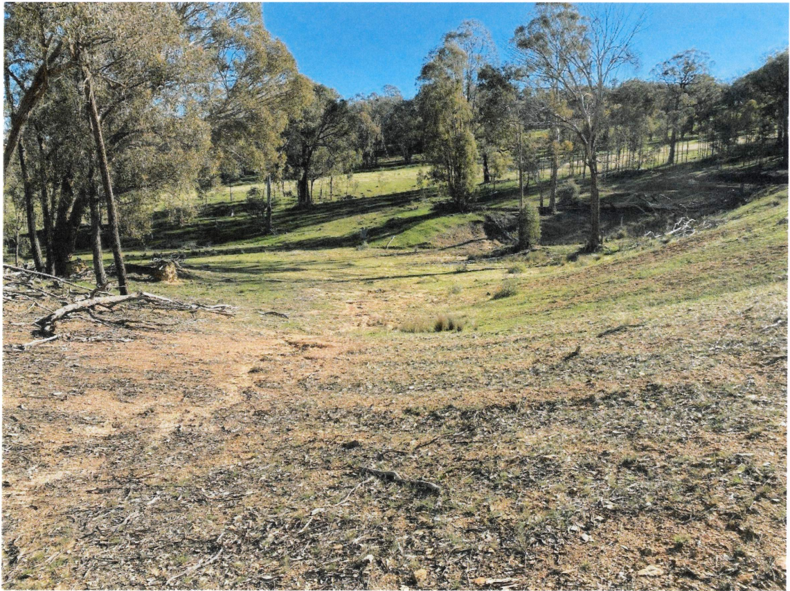
Photograph 6: Minor erosion due to overland flow from southern spillway. Facing West.
