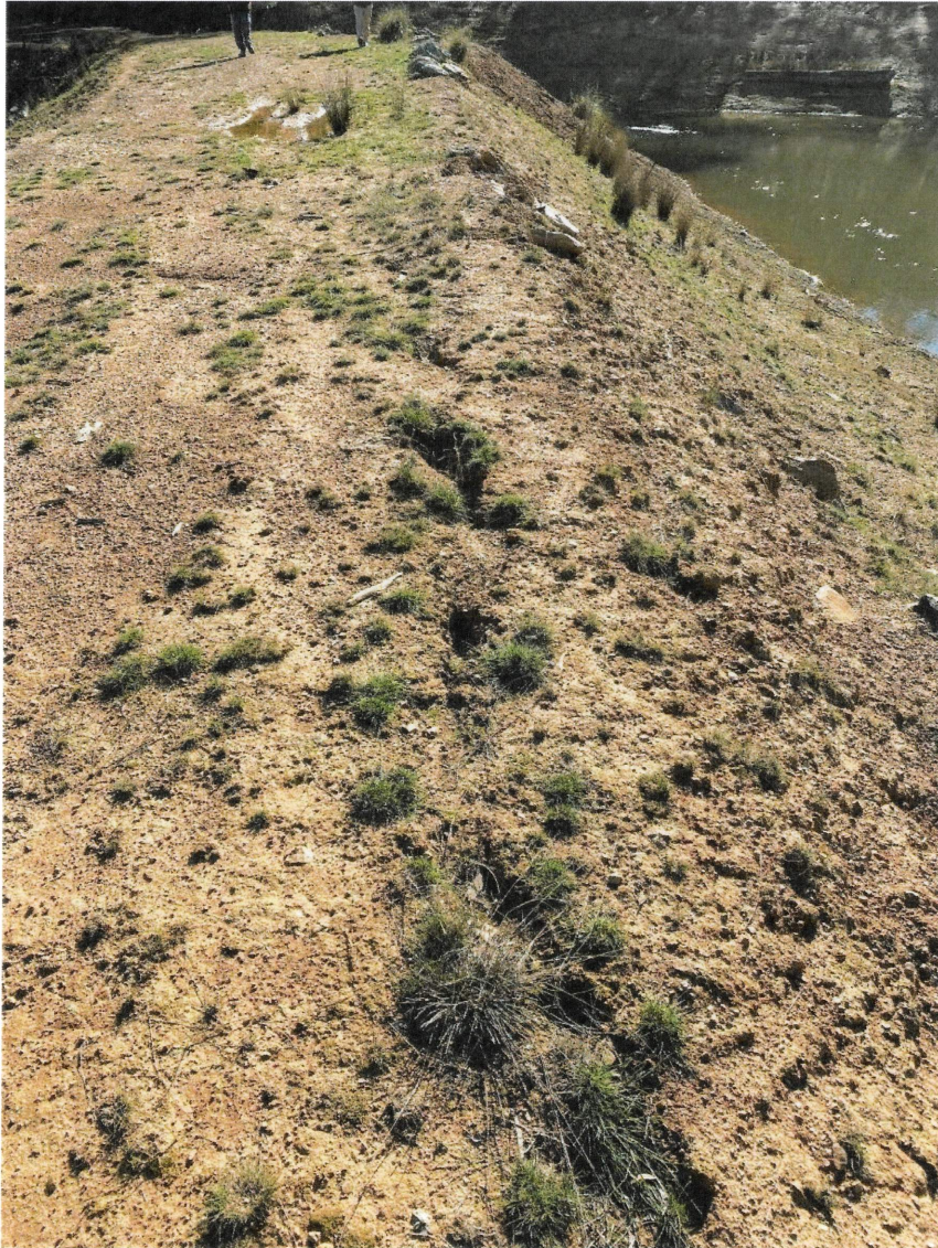
Photograph 10: Tension cracking of eastern side of top of embankment. Facing North.
