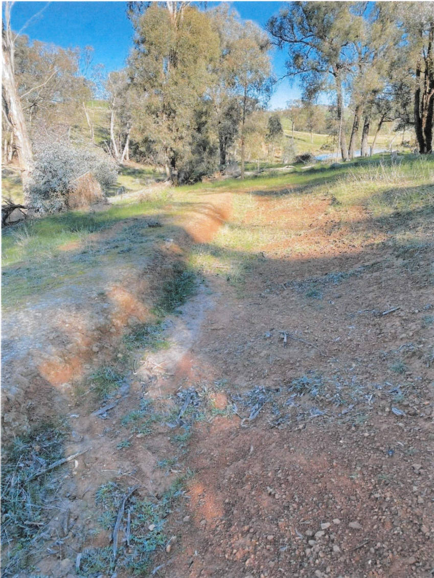
Photograph 21: Northern spillway channel directing overflow from outflow pipe downslope to the west. Facing west.
