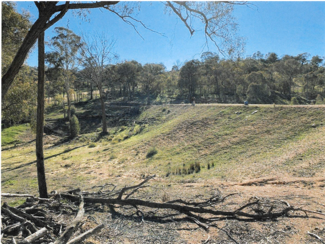
Photograph 5: Dam embankment. Facing North. Minor erosion evident in foreground due to overland flow from southern spillway.
