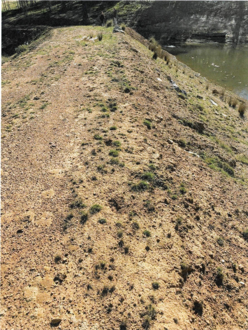
Photograph 8: Evidence of tension cracking along eastern side of top of dam embankment. Facing North.
