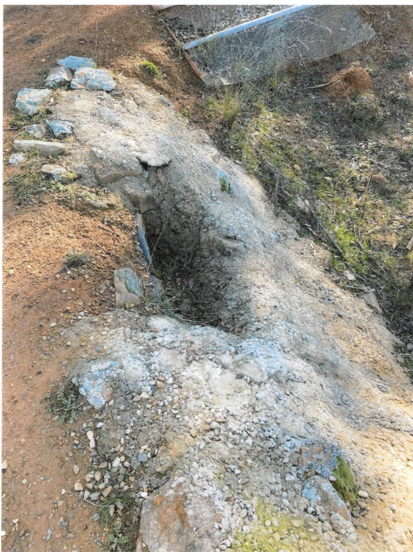
Photograph 19: Spillway with concrete surrounding outflow pipe. Concrete height approximately level with midsection of outflow pipe.
