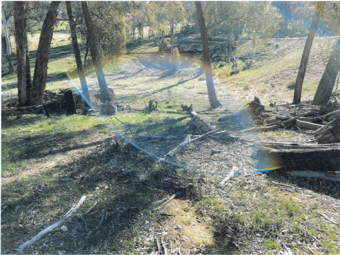
Photograph 4: Minor erosion evident from overland flow of southern spillway. Facing North.
